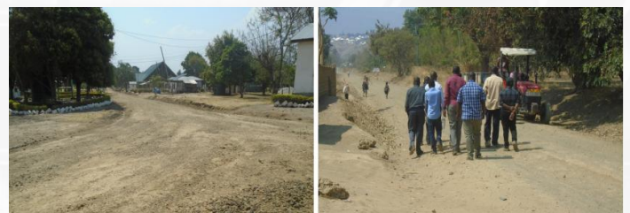
Plate 1: Surface layer of blended cinder, pozzolan and clay materials
