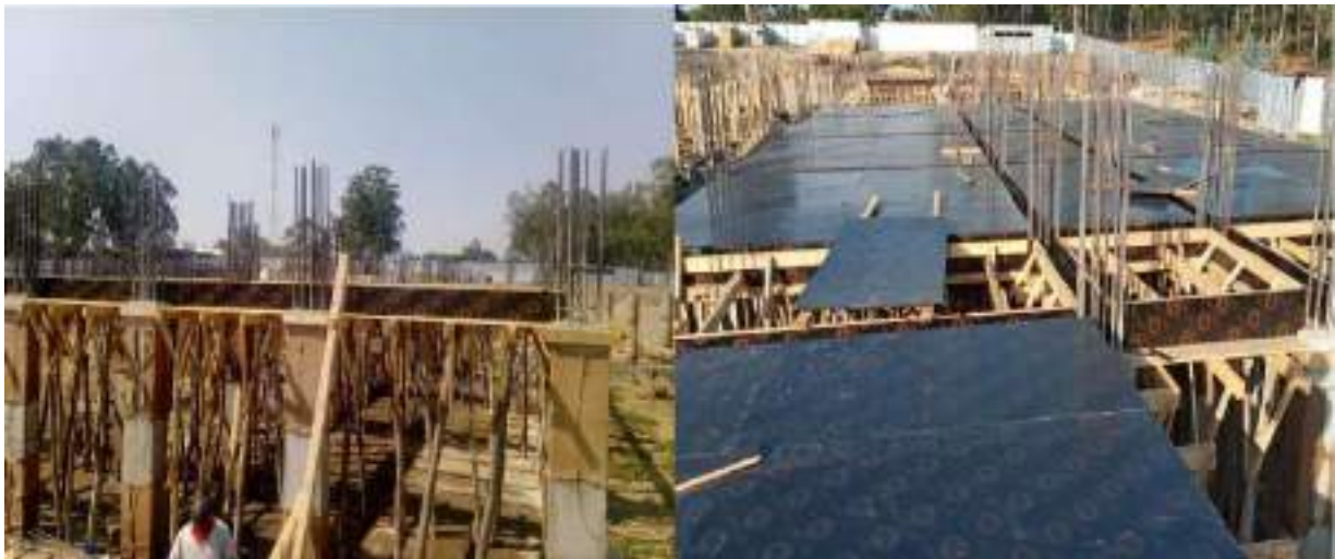
Figure 18: Civil works on reinforcement for beams and slabs including spacer blocks
