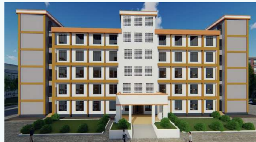
Appearance of MUST Main Campus student's hostel building on completion
