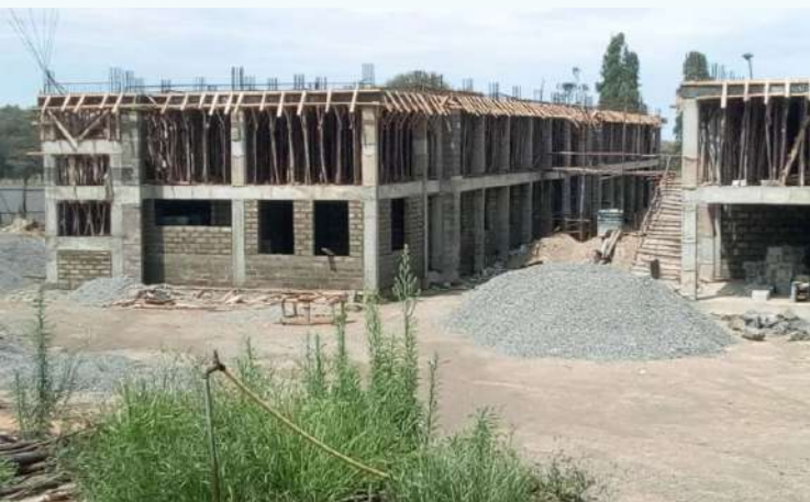
The appearance of MUST student's hostel building under construction
